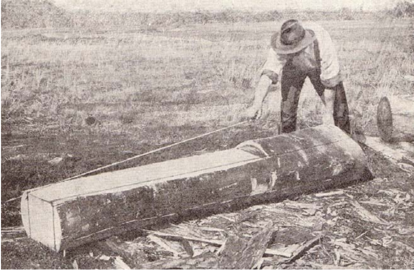
Striking after the first two edges have been squared
