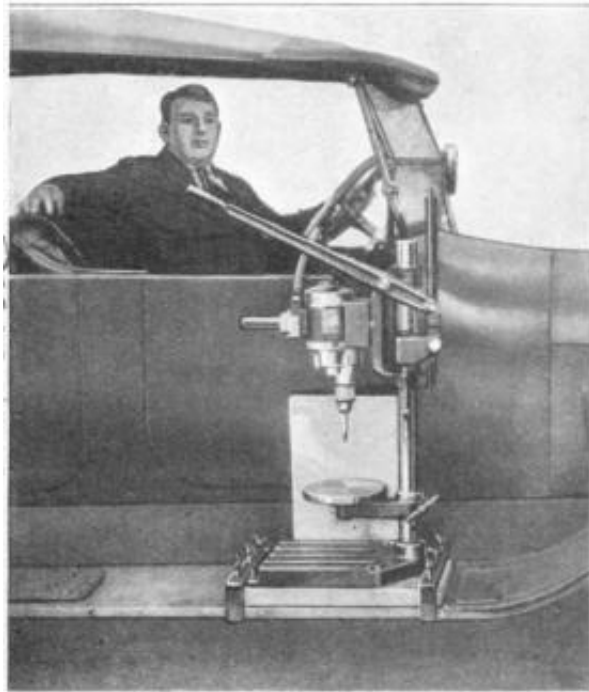
This Drill Stand Holding a Portable Electric Drill was Placed on a Salesman's Car for Demonstrating Purposes
