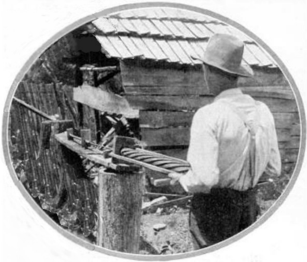
RIFLING. . . Above, the last step in the making of the gun barrel. A spiral-cut piece of wood is used as the guide for the cutter. By pushing the handle back and forth, the smith makes the twisted grooves that insure the accurate flight of the bullet. The cutting edge of the rifling tool is raised as the cut deepens by placing a piece of paper between it and the wooden holder, until the groove has been given the desired depth
