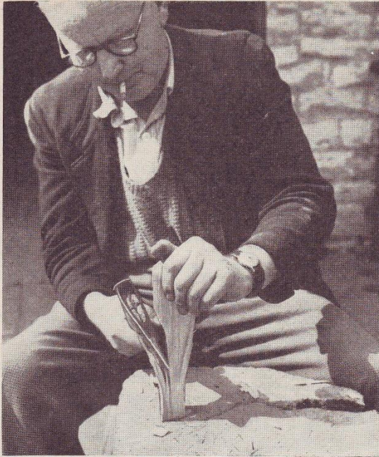
FIG. 1. SHAPING SHOULDERS WITH AXE
