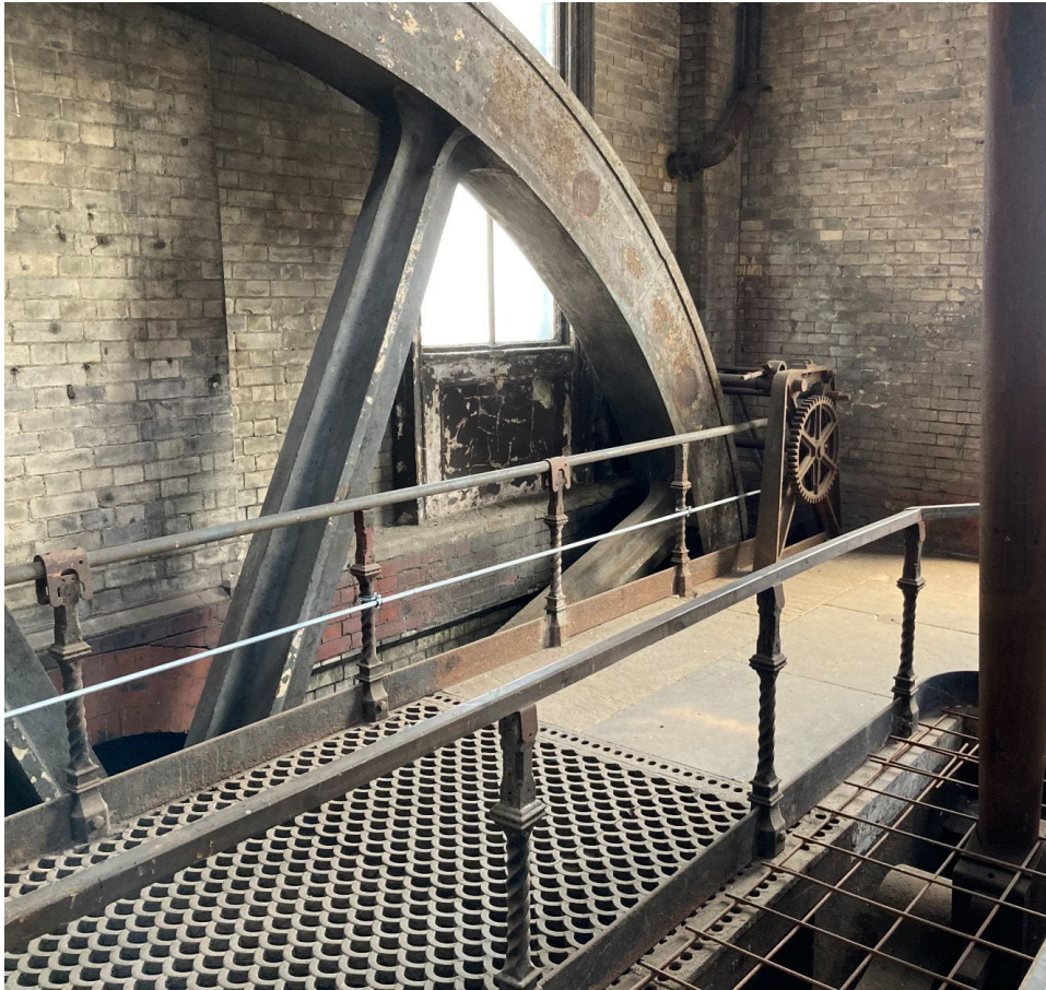
The flywheel pictured above weighs 52 tons and was cast in four sections.
