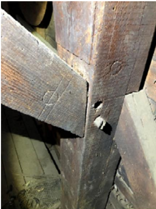
Fig.2. Race knife marks matching a joint in a timber framed building (Marriage Marks). Marks are also found supposedly having the power to avert evil influences or bad luck (apotropaic).
